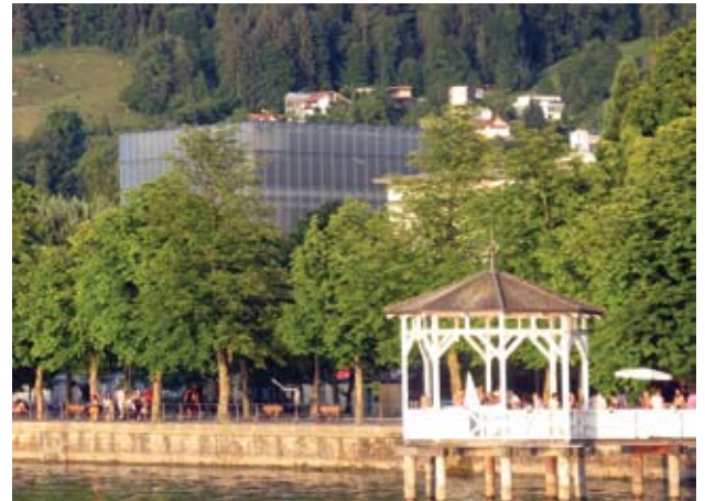
Arh. Peter Zumthor, muzeul din Bregenz, Austria 1998 / Architect Peter Zumthor, Bregenz Museum, Austria, 1998
